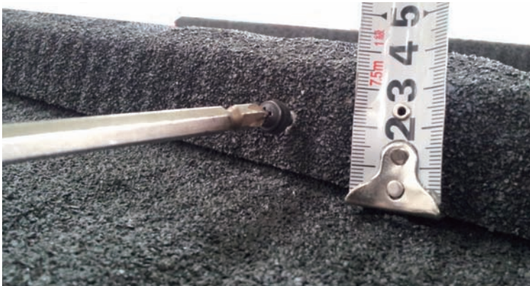
Dimple is easy to install because the up stand part is 35mm wide
